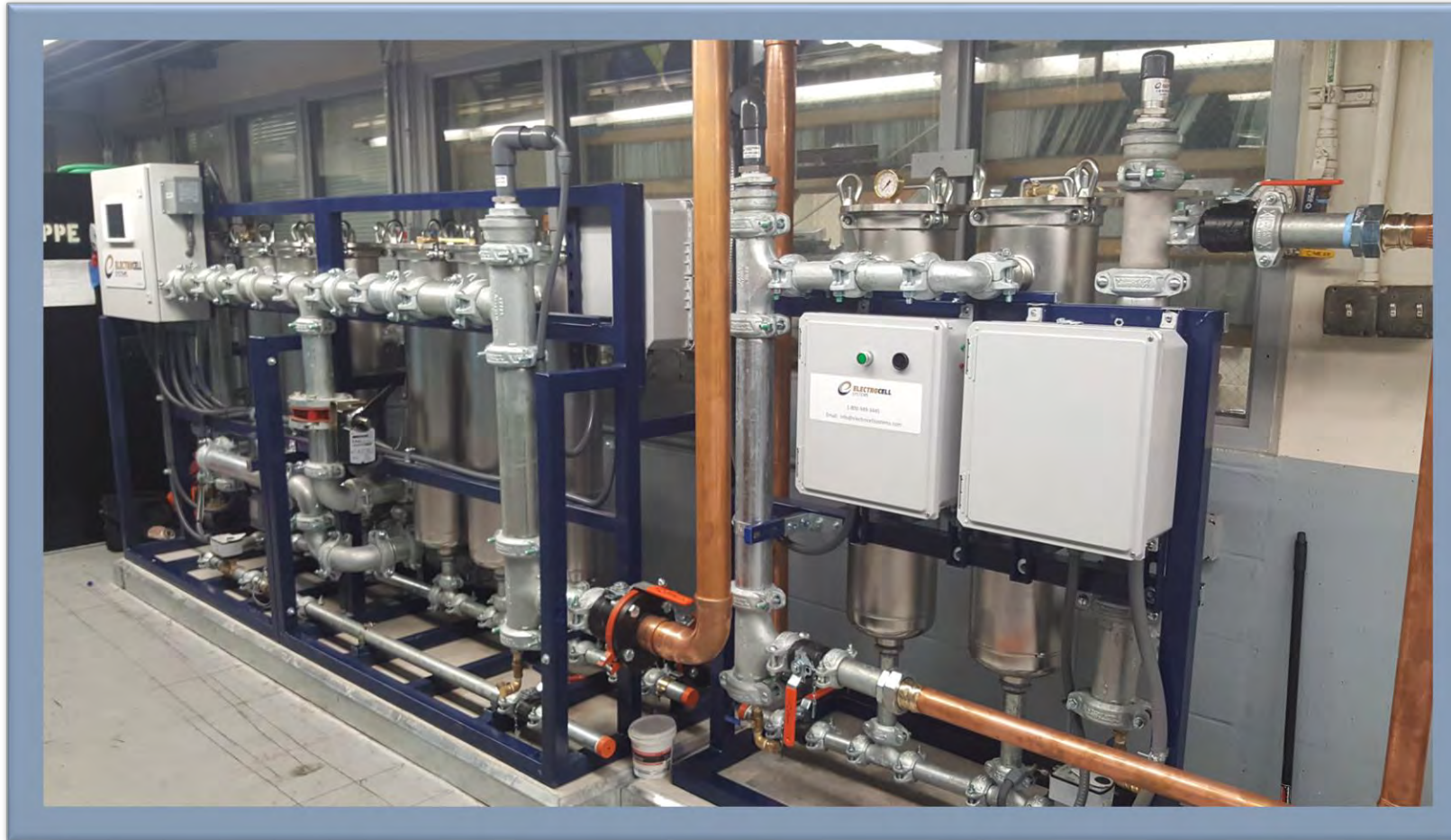
XCell-6000 Precipitator (on Open Loop) paired with the XCell-200-PP (on Closed Loop)
